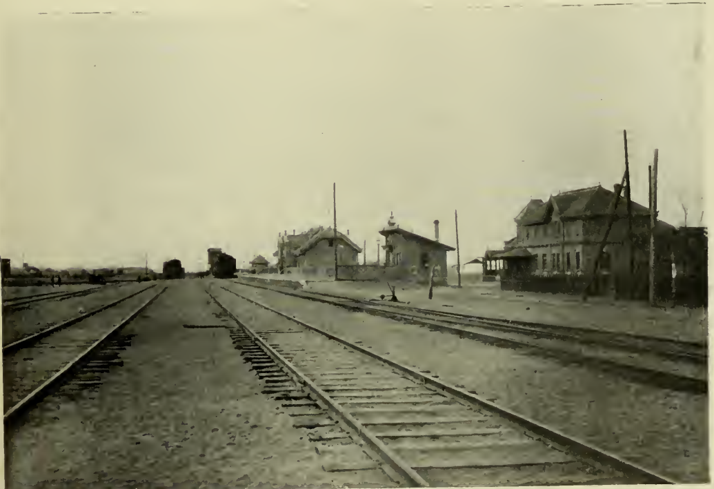
A TYPICAL STATION ON THE MANCHURIAN RAILWAY.
